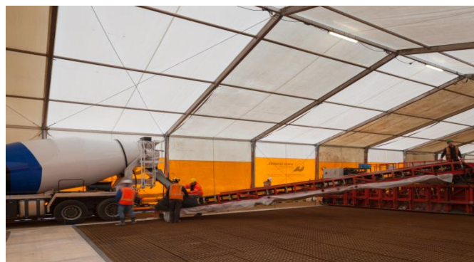
Figure 2: 100 m of bridge slab could be paved in one day. (Photo: Bart van Hoek)
