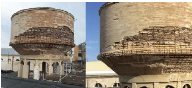
Figure 4: The steel-reinforced concrete of the water reservoir tower in the Grand Harbour region of Malta, to be retrofitted with TRC
